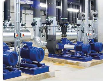
MOTOR CONTROL DEVICES, ETC.
